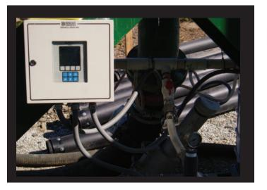
In addition to the 4-20 mA calculated mass flow analog output, the X96 product family may be configured to provide alarm contact closures on various process parameters (Flow, Density, or Mass Flow).
