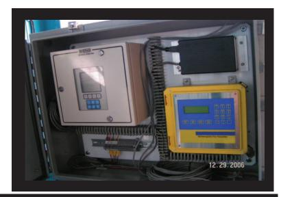
In the block diagram on the front page, the slurry to be monitored is passed through a steel pipe. The gamma source and detector are externally mounted and measure the density of the material flowing through the pipe which may be displayed on the X96 display. A magnetic flow meter is coupled to the pipe to measure the rate of flow of the slurry. The X96 controller accepts the density and flow date to calculate and display the mass flow of the material.
